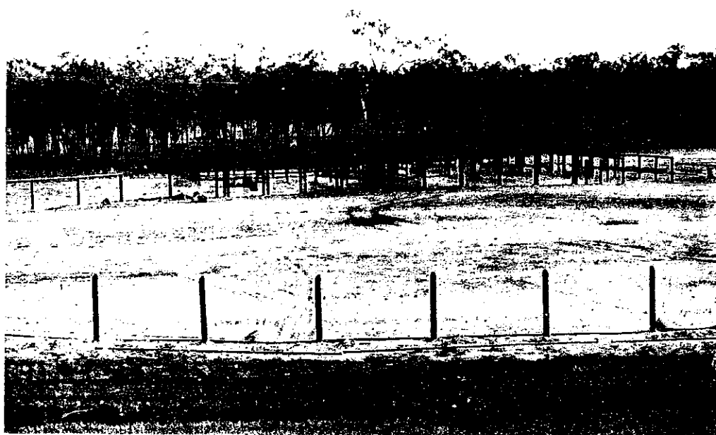
The Moranbah rodeo Ground is a standing example of using second hand materials to good advantage. The entire complex is being constructed from used water pipe and old conveyor belting which normally would have been discarded. The first rodeo should be held at the new grounds in June. People interested in helping with construction are asked to call Dave Ethel on 507 373. The Moranbah grounds were designed by Dave, who has had many years of experience with rodeos throughout most of Australia.
